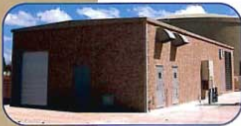
30' x 70' Pump Station.
