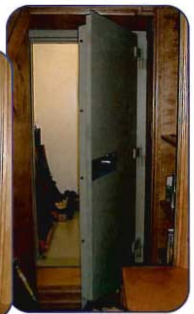
Fire rated tornado vault installed on house slab prior to construction.
