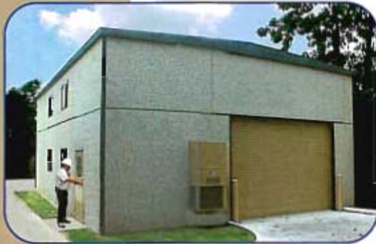
30' x 40' x 16' Pre - engineered operations building.
