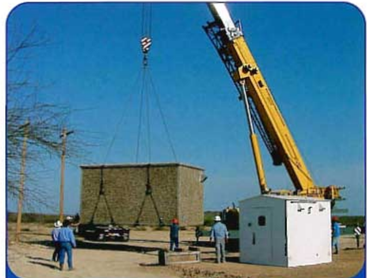
Complete Turnkey 12'x20'x10' Chemical Control Building. Buildings up to 14'x24' can be shipped fully assembled. All electrical and hardware for your process can be preinstalled in a concrete building ready for your jobsite.
